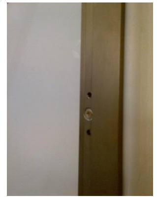
Securing and fastening the wall profile by counterboring the countersunk holes in the profile into the wall and impact screw fastening.
