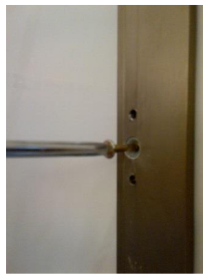
Securing and fastening the wall profile by counterboring the countersunk holes in the profile into the wall and impact screw fastening.
